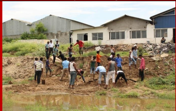
Desilting of Pond
