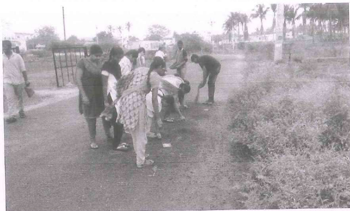
Road repairing work from Veppampalayam to College on 26.09.2017
