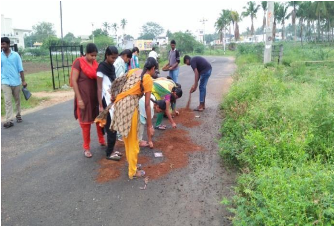
Road Repairing Work to Public
