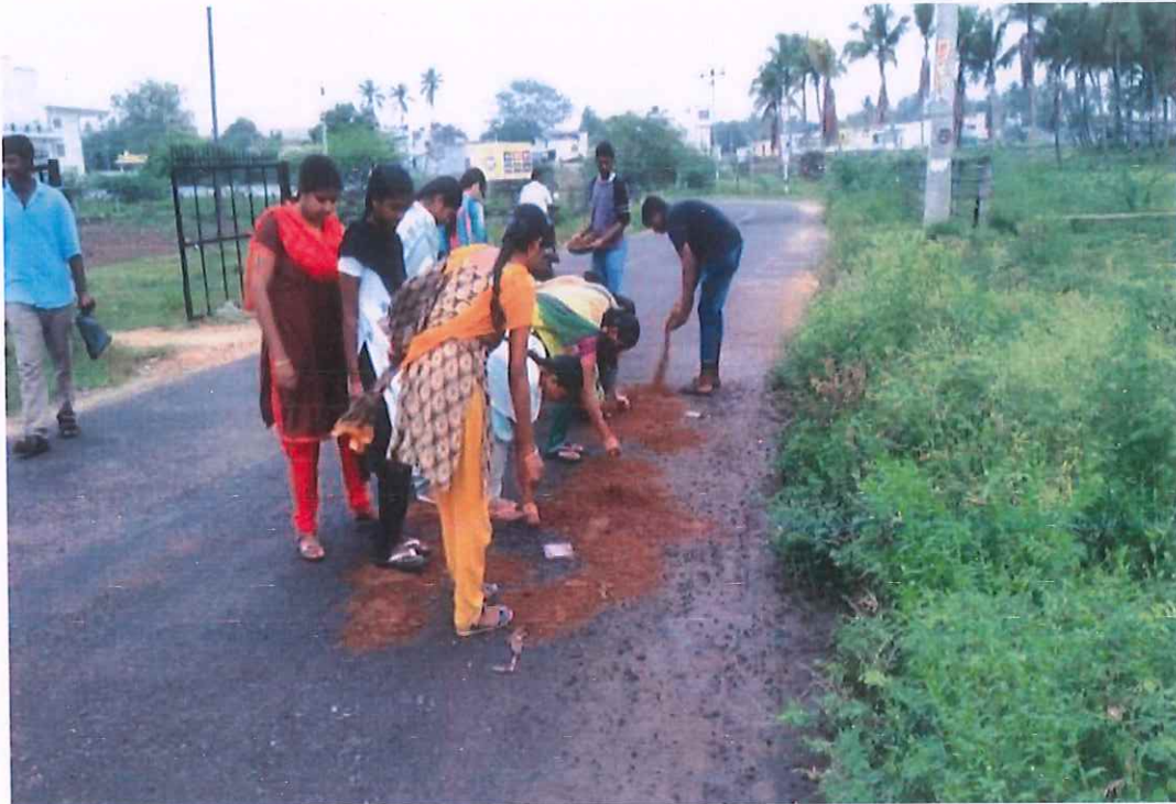
Road Repairing Work to Public
