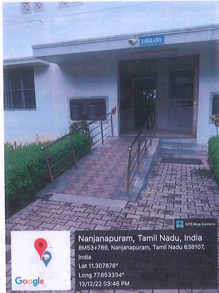
Ramps & Rails Located at Library Entrance
