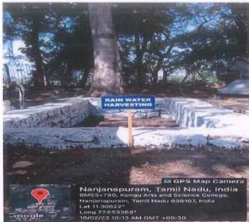
Rainwater Harvesting pit at Fitness Centre front side
