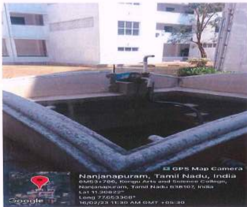
Overall Collection tank at main block
