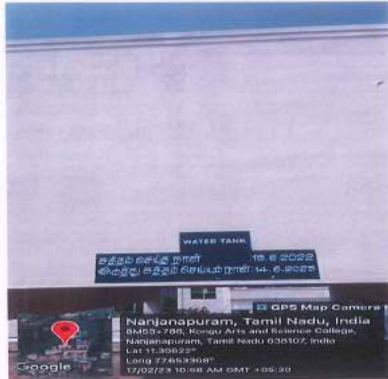
Overhead Ordinary Water Tank on the terrace of PG block
