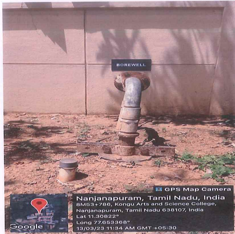
Borewell near the Principal Quarters
