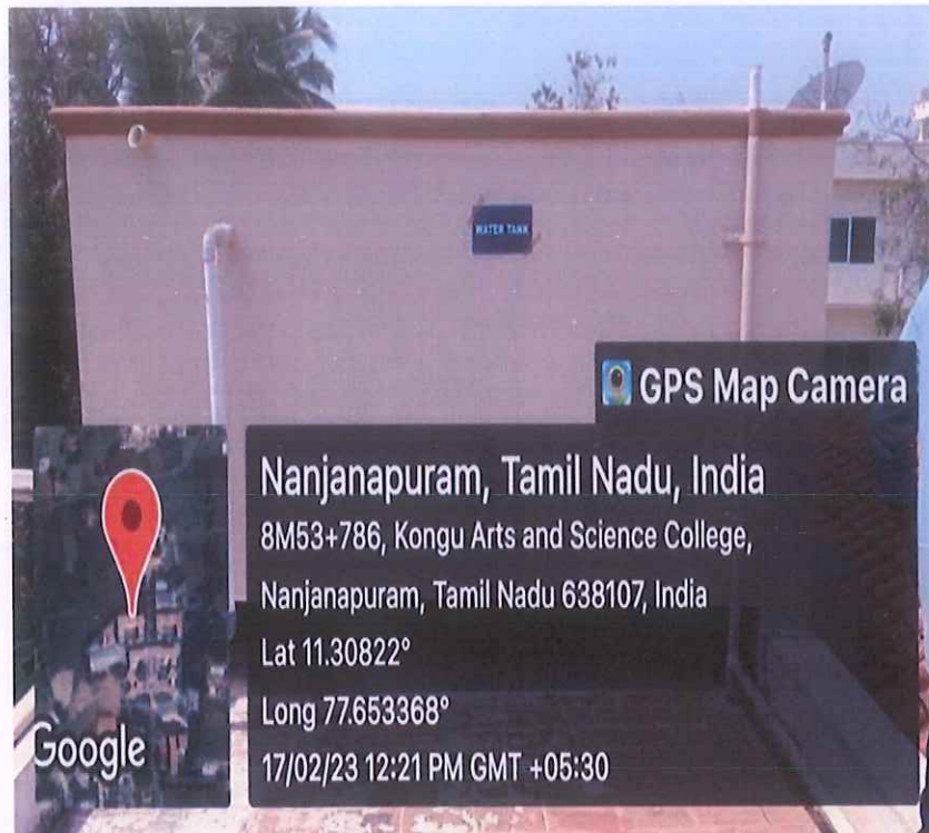
Overhead Water Tank on the terrace of principal quarters
