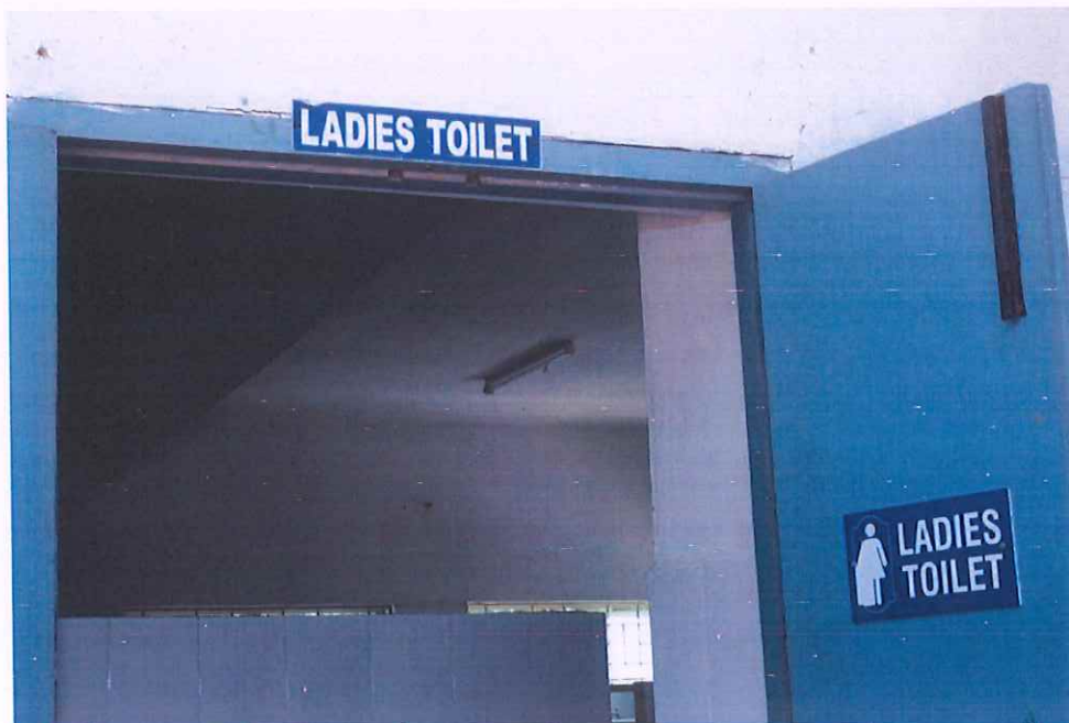
LADIES WASH ROOM AREA
