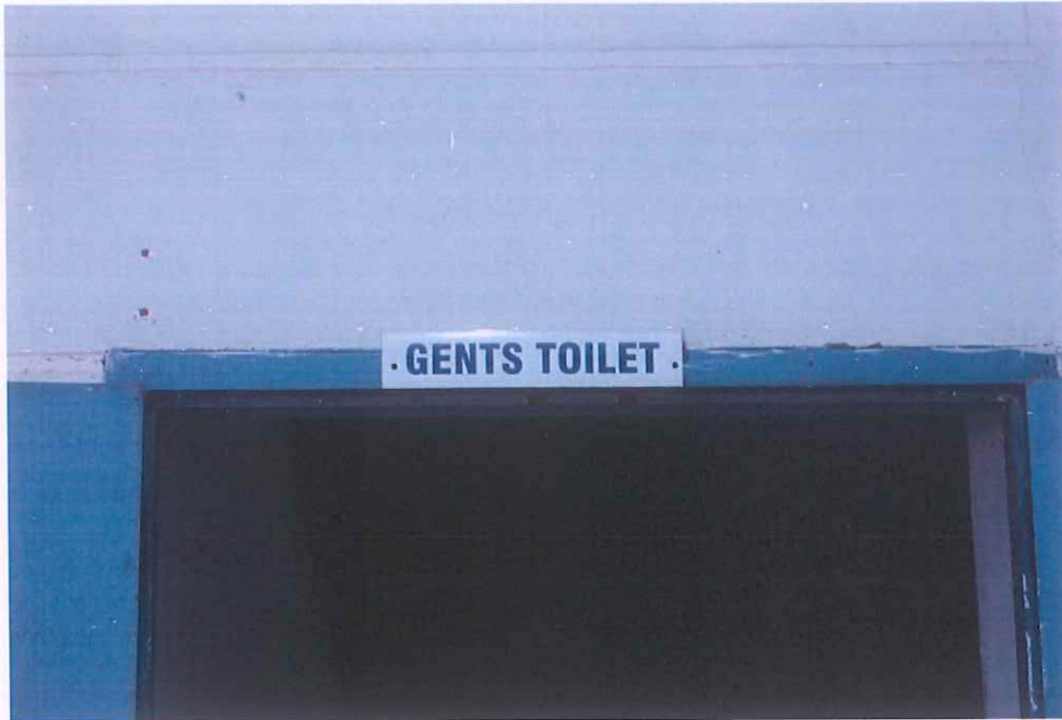
GENTS WASH ROOM AREA
