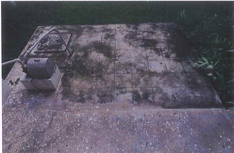
GROUND WATER TANK STORAGE AREA
